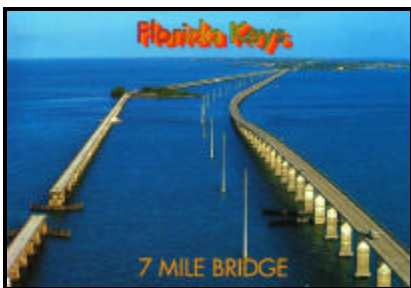
The Seven Mile Bridge. Note the old bridge on the left. Bigger.
